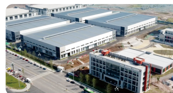
Yibin Industrial Park
