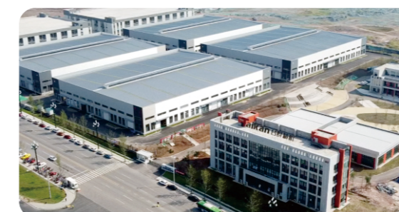
Yibin Industrial Park
